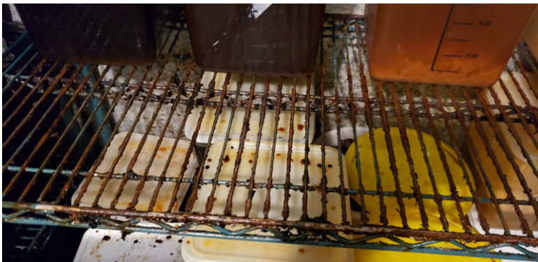
Rusty shelves in walk-in cooler and flakes of rust on food containers
